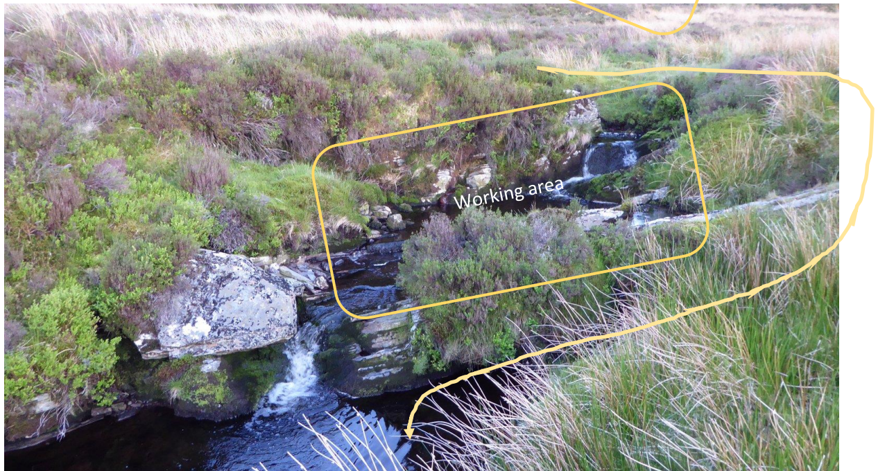
Figure 3 (a, b) Syphon route past working area.
