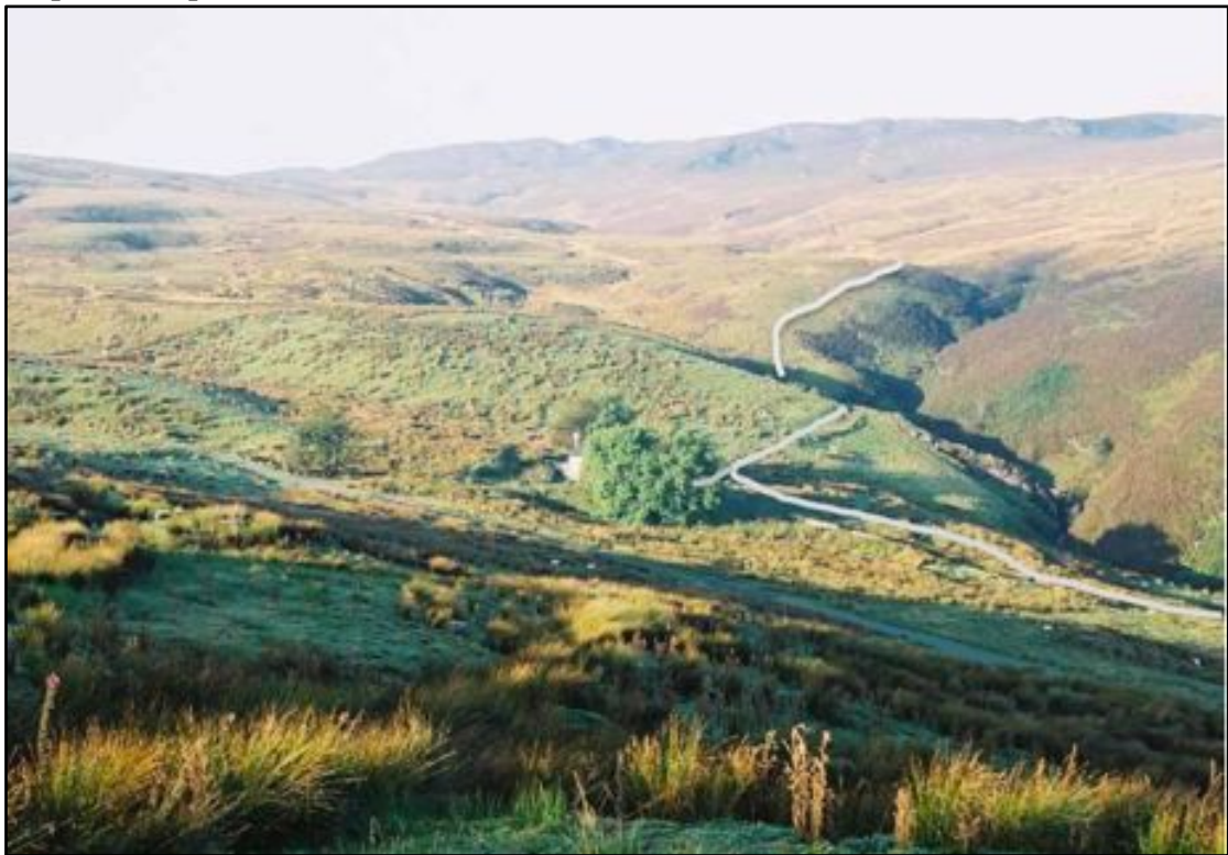
Map 2: The upper section of the penstock to show the T-off for the water supply to the house (behind trees).
