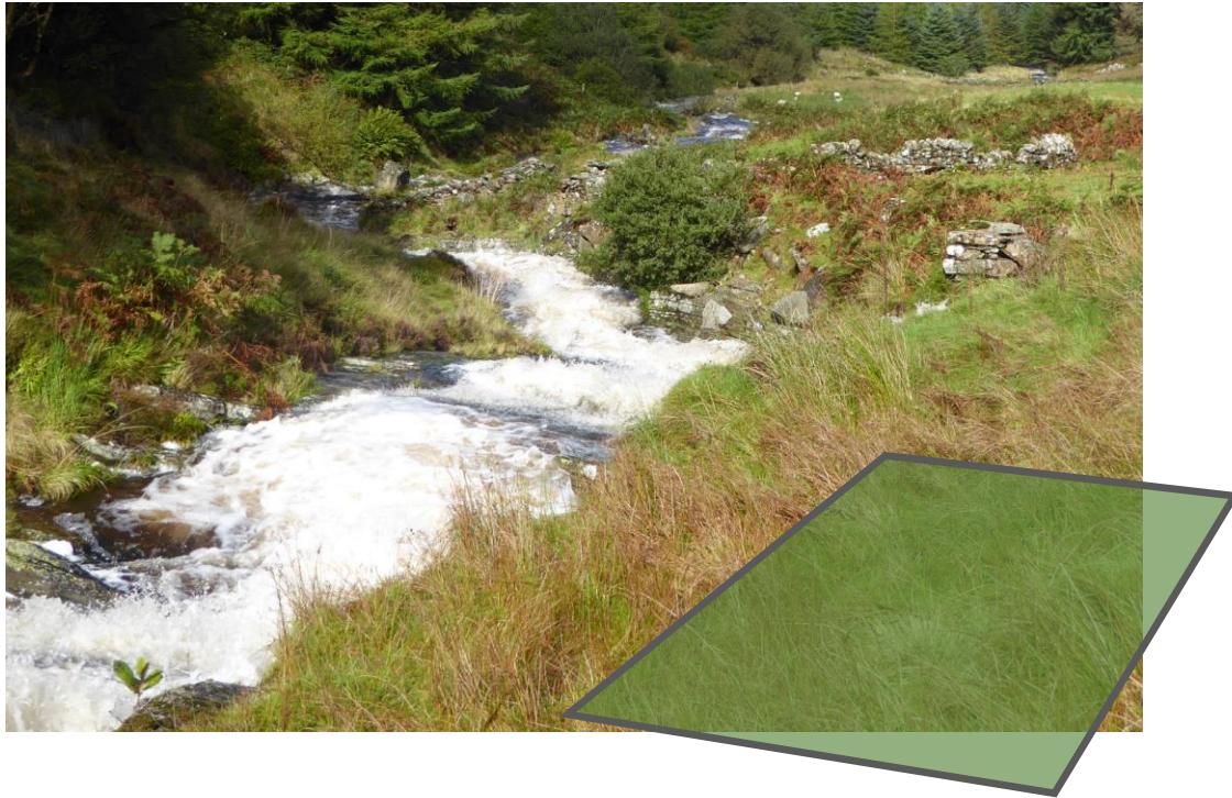
Figure 22. Turbine hut location after very heavy rain (15 th September 2017). It does not flood.
