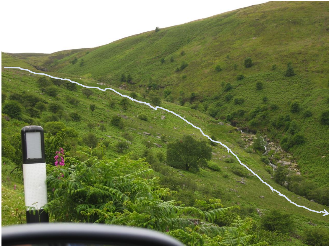
Figure 6. Pipe route below house.
