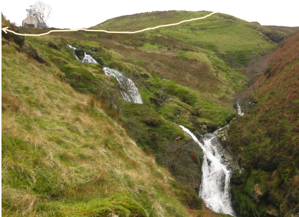
Figure 4. Pipe route past cottage.
