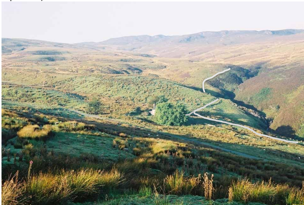
Figure 5. The penstock has a tee-off to the house before continuing for another 475m towards the bottom of the valley.
