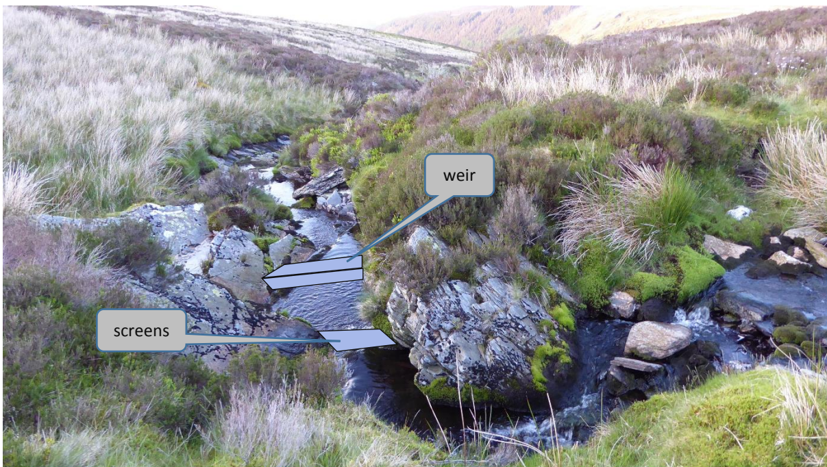
Figure 12. From close-up, the extraction system will be hidden down between the stream banks.
