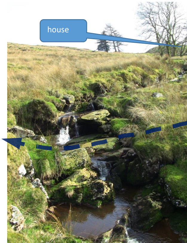
Figure 9. Second crossing point. The pipe will have a small air-release valve near each crossing point. The air valves will be provided with a conduit so that if they ever leak, any water returns to the stream and cannot not erode the surrounding soil.
