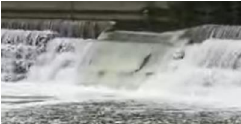
Figure 24. Brown trout swimming up a weir ( https://www.youtube.com/watch?v=tMvexb97TqA ). The flow in this video separates from the edge of an inclined flat plate. The fish find it difficult to get past the lip, especially at this low flow condition which leads to a rapid change in gradient at the lip. An ogee profile with attached flow should be easier to traverse.
